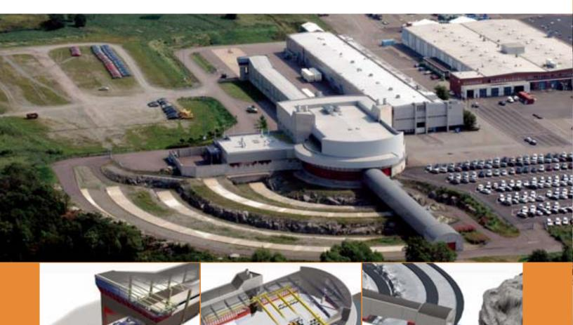
This fixed test tunnel is used for collision tests inside the center, and for rollover tests outdoors.
